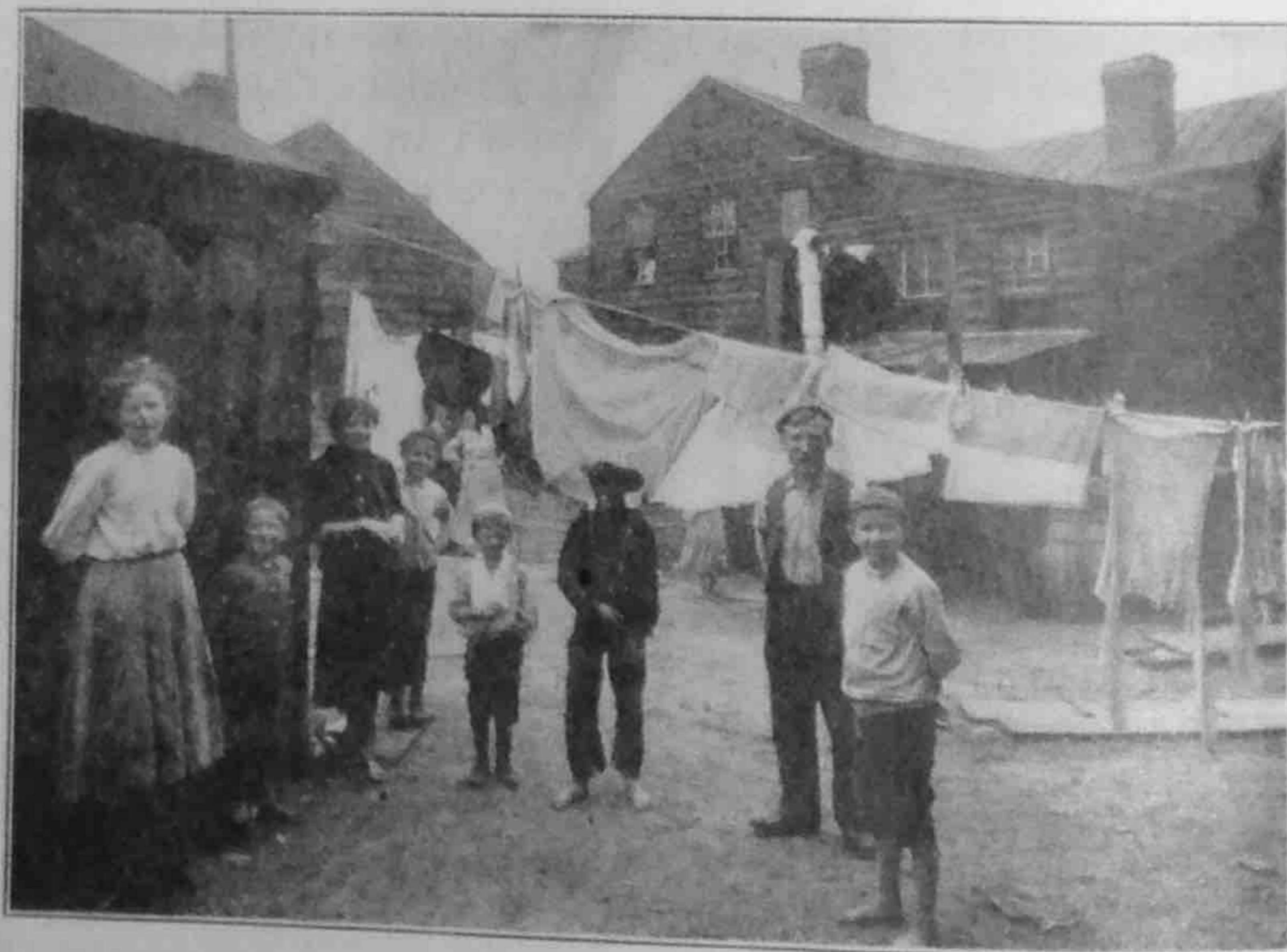
STEEL WORKERS—BETHLEHEM, PA.
